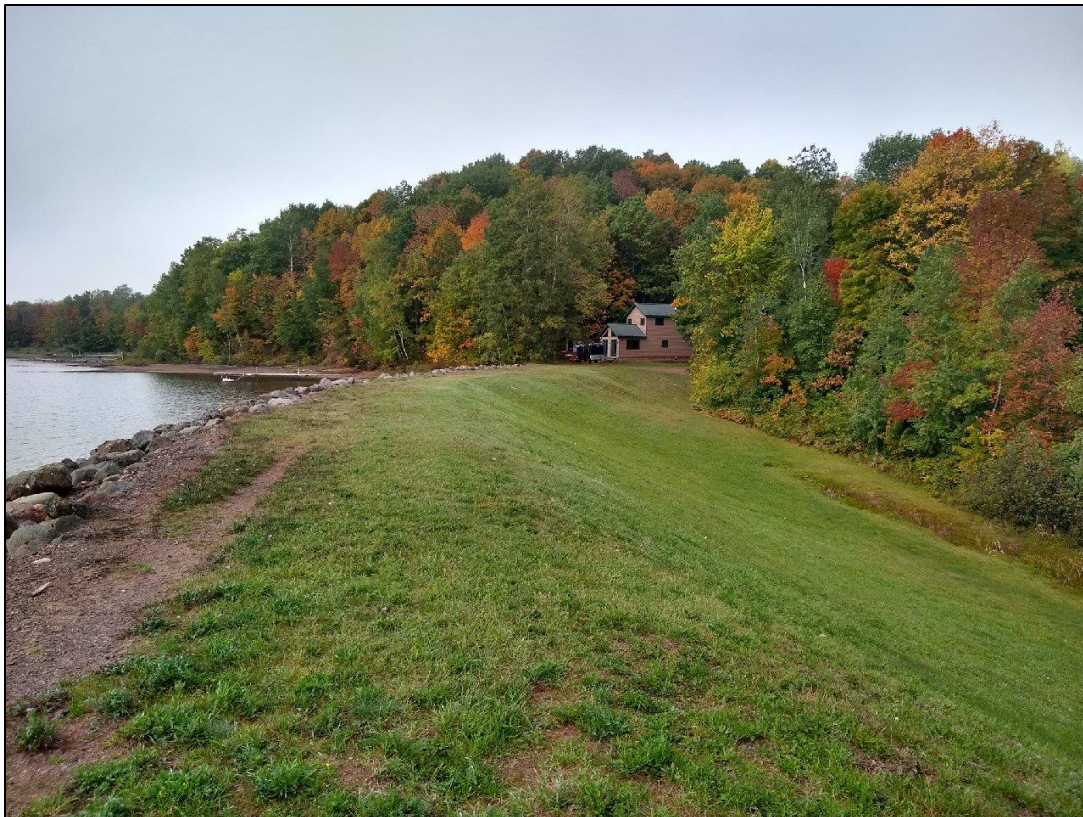
Figure 3.10.1-2 View of Gile Dam Looking West
